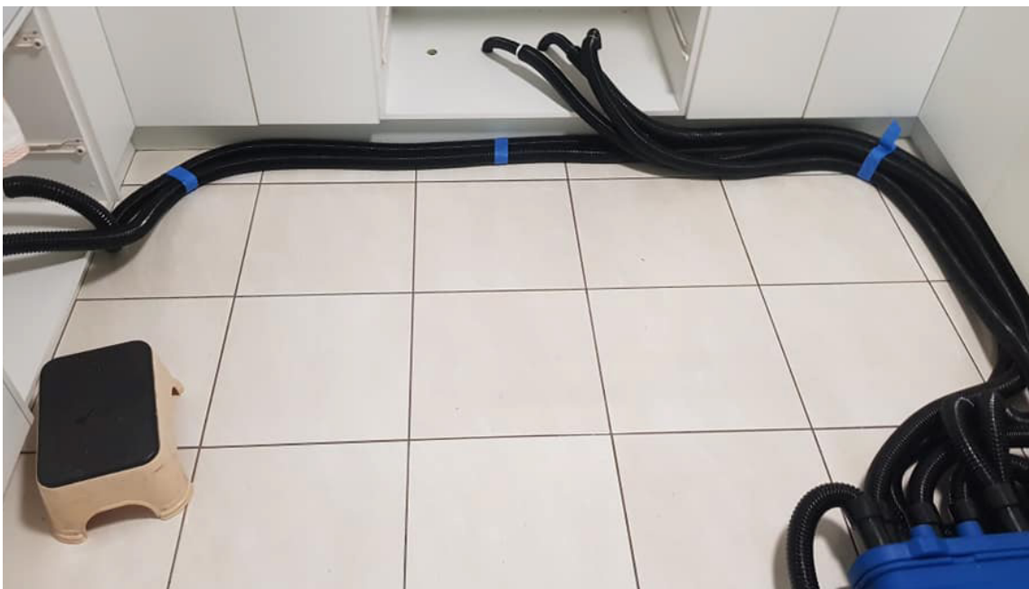
Example: Kitchen Cabinetry Drying - Using the 38mm to 25mm Reducers (Kitchen Kit)
