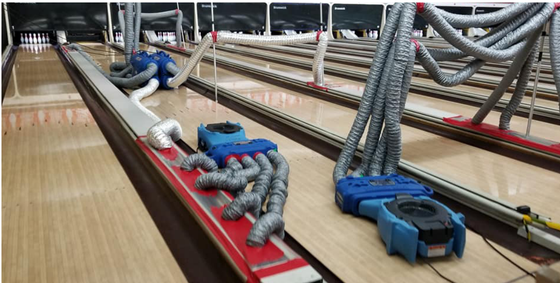
Example: Target Drying of a Subfloor Space
